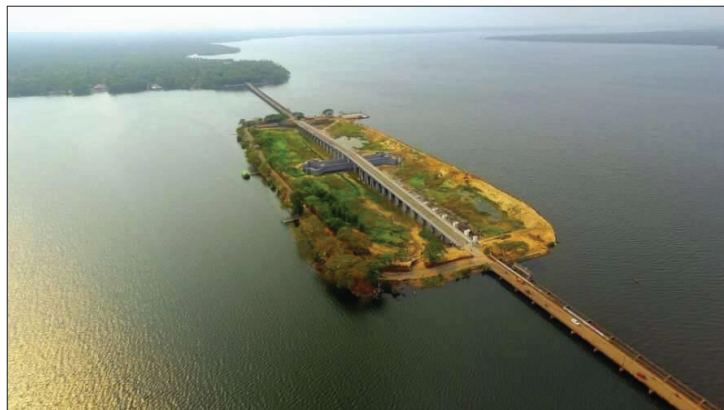
Figure 6 : View of Thanneermukkom barrage
