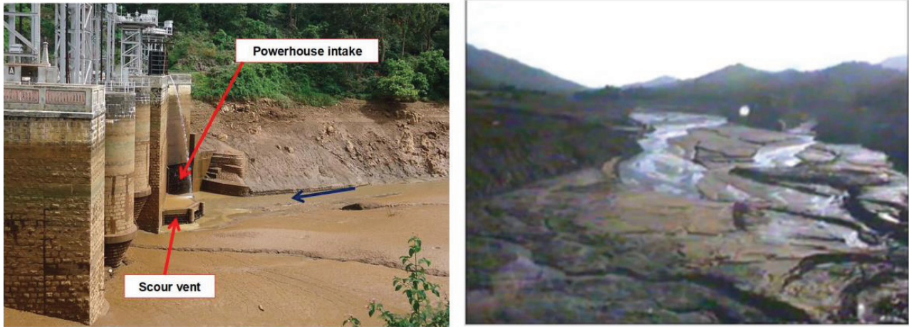
Figure 2 : Deposition in the Kunda Palam (left) and Pillur (right) reservoirs during depletion in 2015 and 1992 respectively
