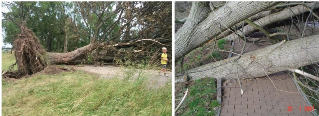
Figure 8 : Tree failures at levees as a cause of strong storm events after a storm 2014 (left) (Source: SEB Düs-seldorf) and 2007 (right) (Source: LUA Brandenburg).
