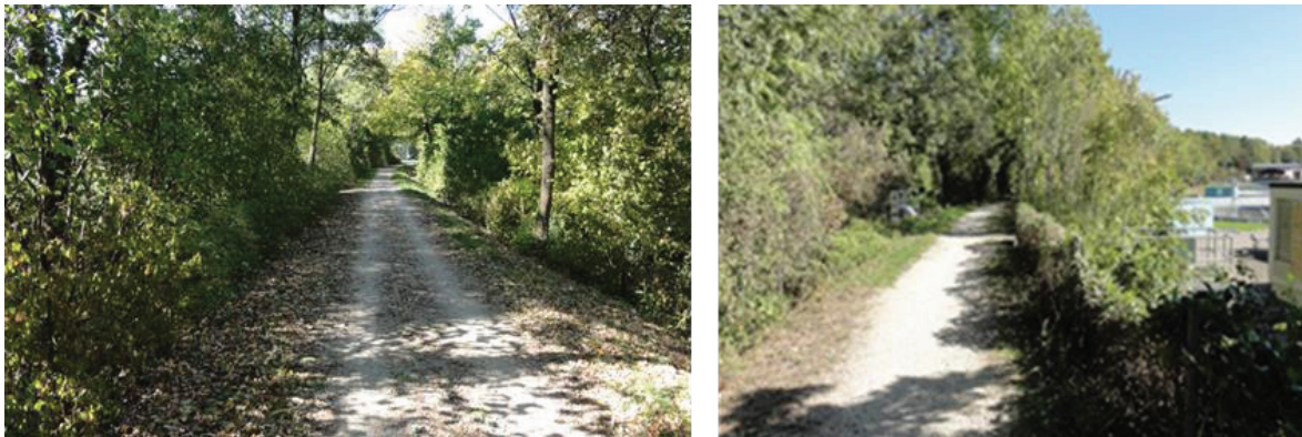
Figure 13 : Existing levees along the Neckar River at the city of Nuertingen with large trees on both slopes (taken from Kerres & Haselsteiner, 2018).
