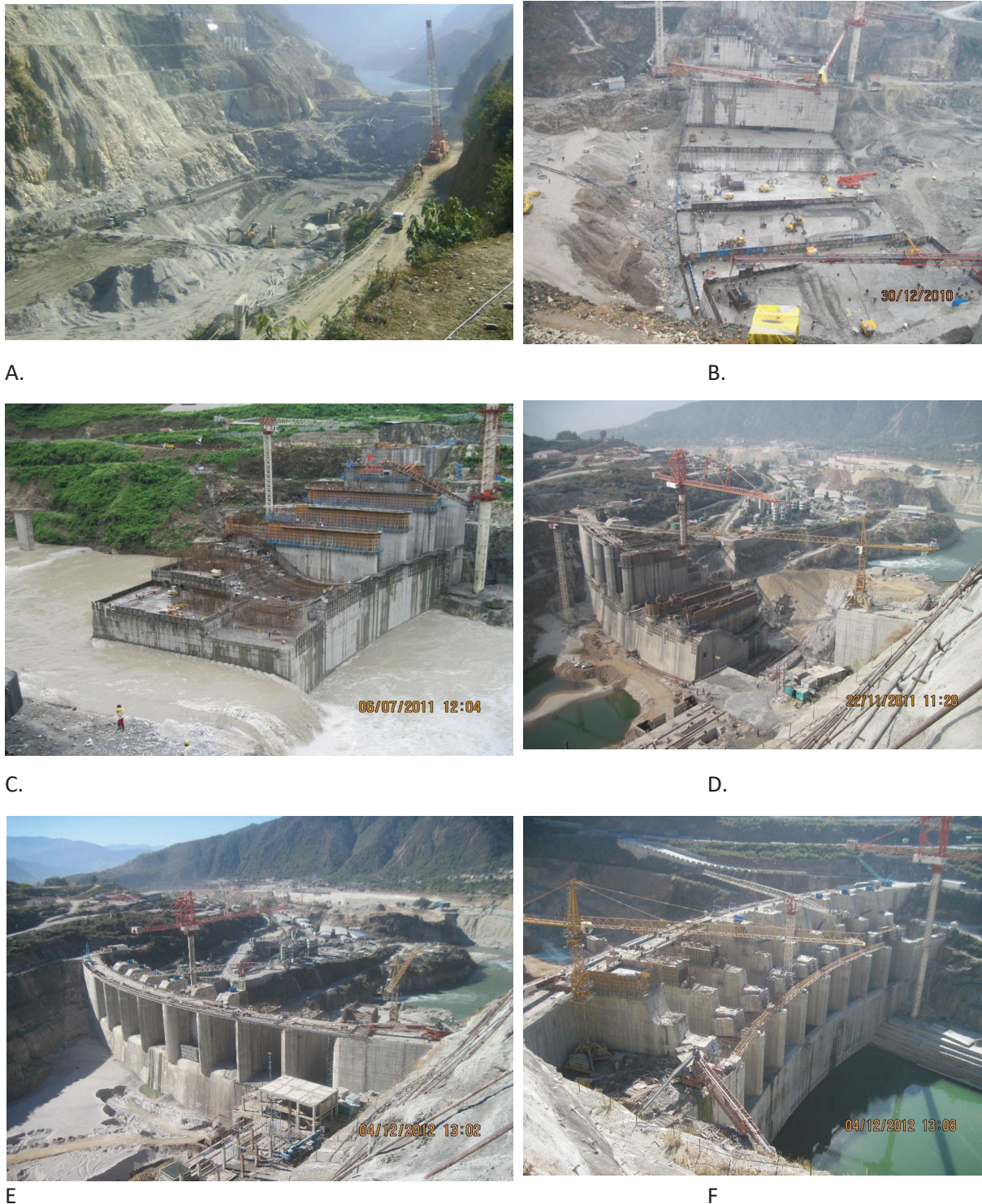
Figure 2 : Construction Phases of Srinagar Dam,
