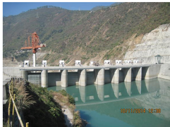
Figure 5 : Dam after Reservoir Filling
