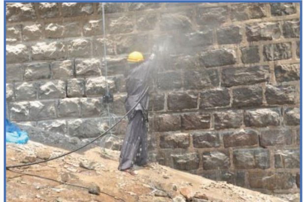
Figure 5 : Surface Preparation (Water Jet)- During Execution
