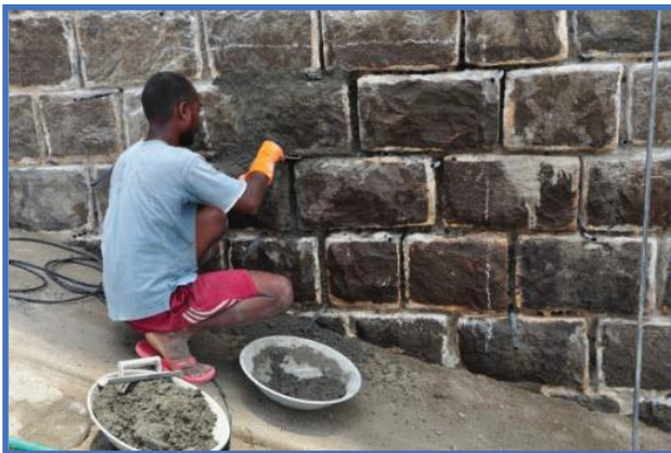
Figure 6 : Application of cavity Filling- During Execution
