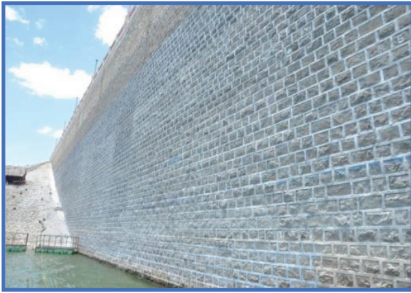
Figure 11 : Epoxy Pointing Coat- During Execution
