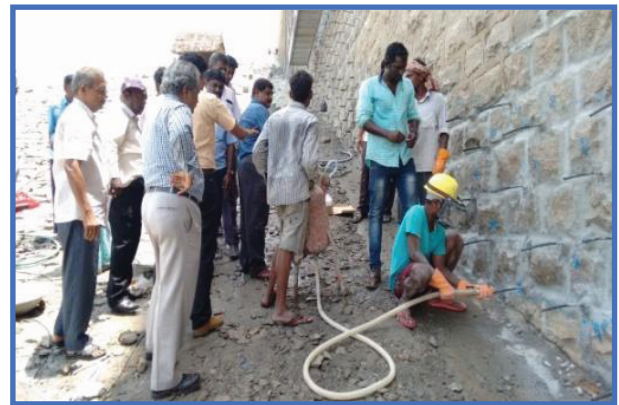
Figure 8 : PVC Nozzle Insertion- During Execution
