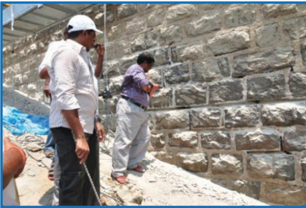
Figure 4 : Surface Preparation- During Execution
