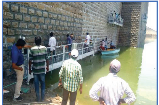
Figure 6 : Application of cavity Filling- During Execution
