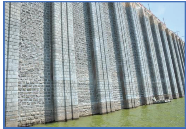
Figure 12 : Application of Pointing Mortar- During Execution
