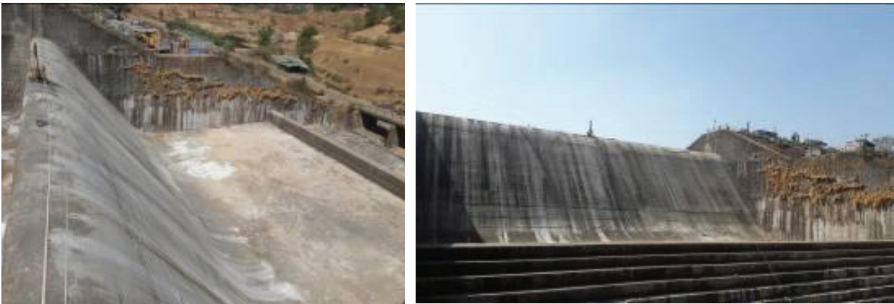
Fig. 12 & 13 : View from top and d/s of Domihira dam after Grouting
