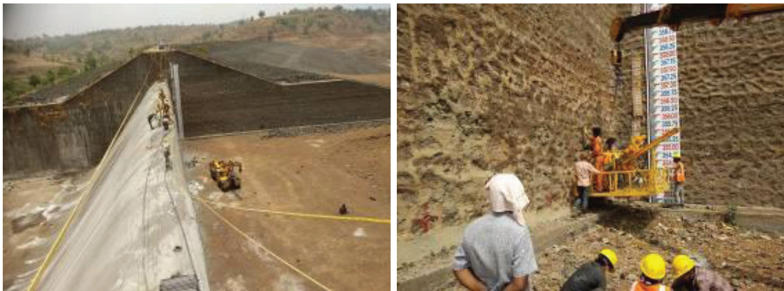
Fig. 9 & 10 : Grouting in Progress in Domihira dam
