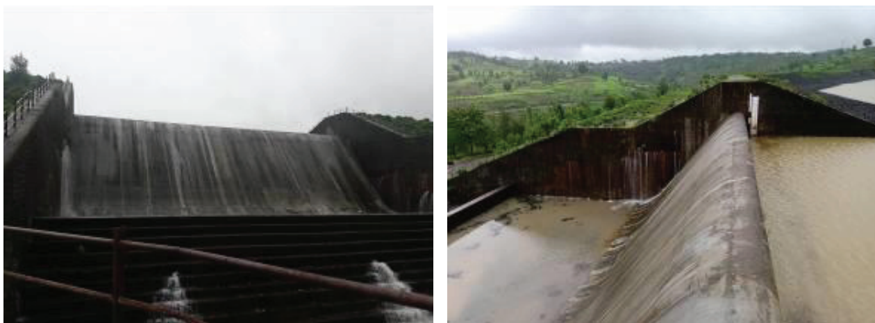
Fig. 14 & 15 : View of spillway after grouting.
