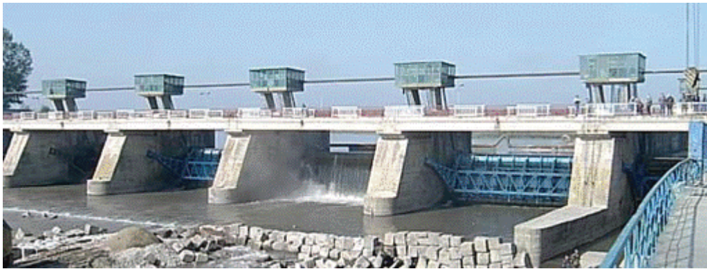
Figure 1 : Downstream view of Isalnita Dam
