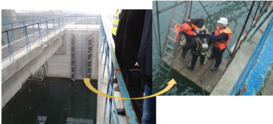
Figure 4 : New stoplog guidance
