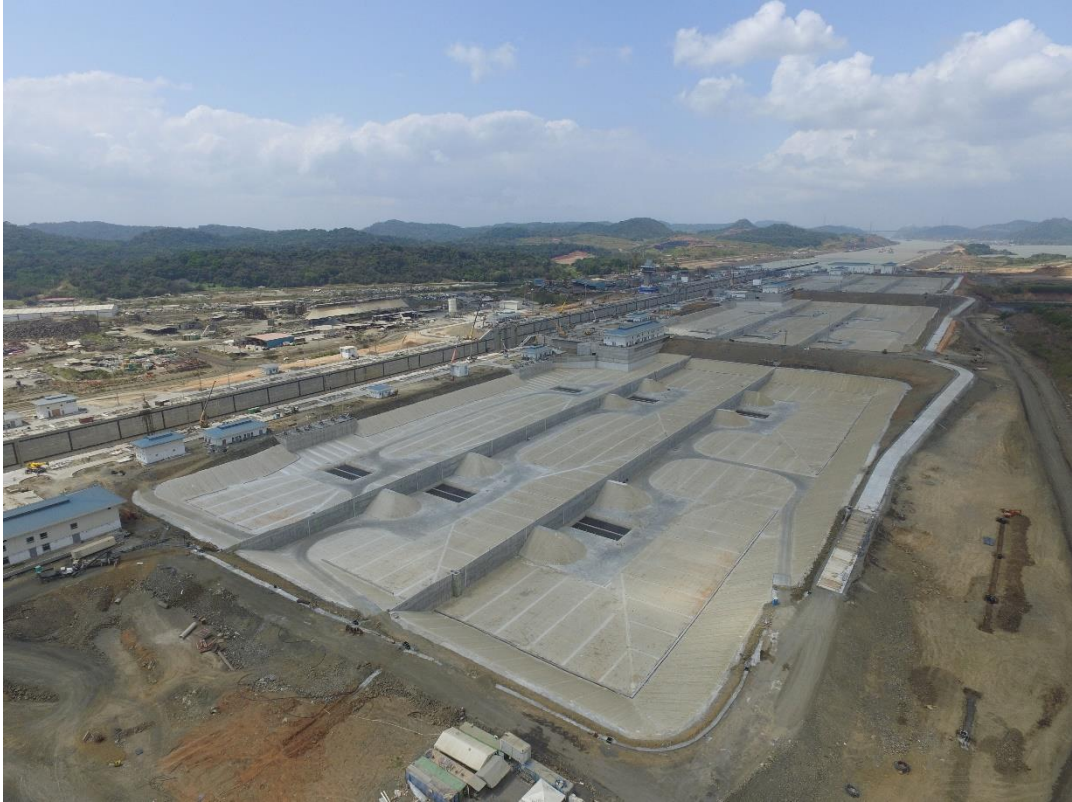
Figure 1: New Panama Canal (courtesy from Carpi)
