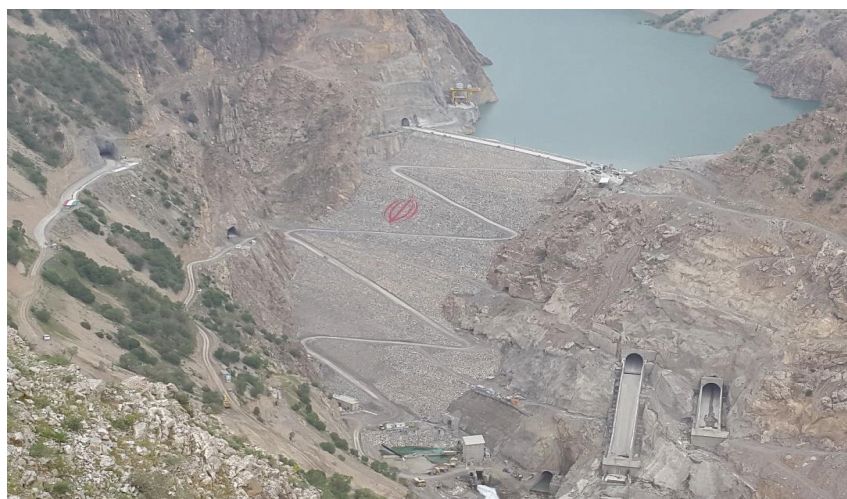
Figure 1 : Downstream view of Rudbar Lorestan ECRD and the two tunnel spillways on the left abutment.
