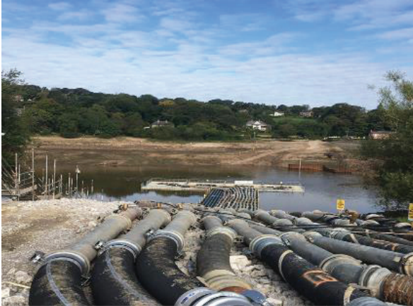
Picture 14 : Pumps on Pontoons
