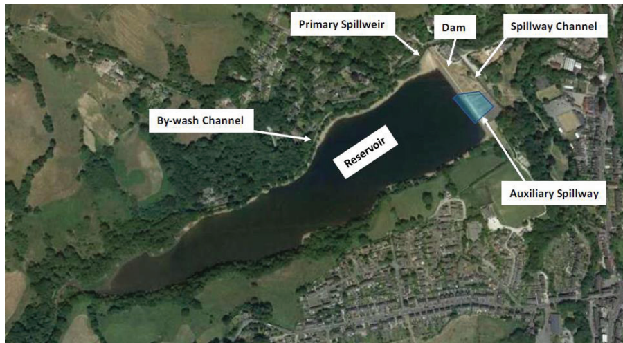
Picture 3 – The Layout at Toddbrook Reservoir
