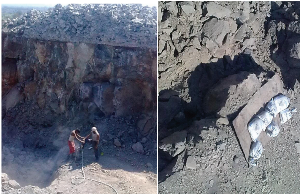
Figure 7 : Photographs showing drilling and blasting operations at Yedgaon Dam site
