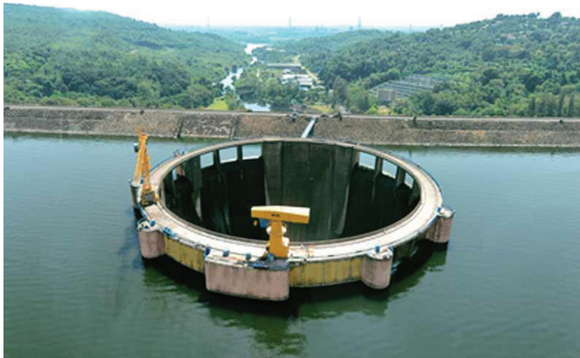
Figure 1 : Ir. H. Djuanda Dam
