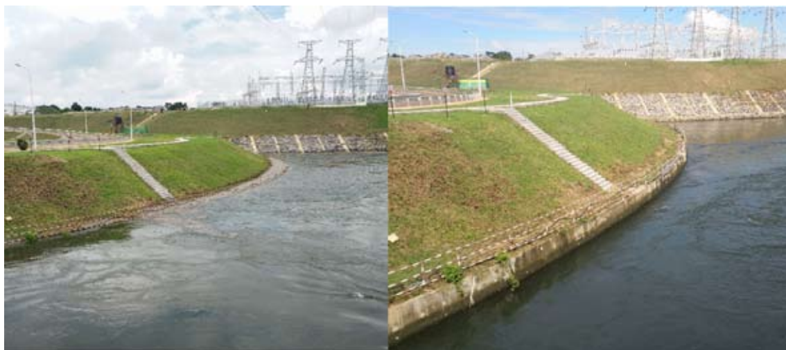
Figure 10 : Showing the downstream water levels during the test and after reinstatement process
