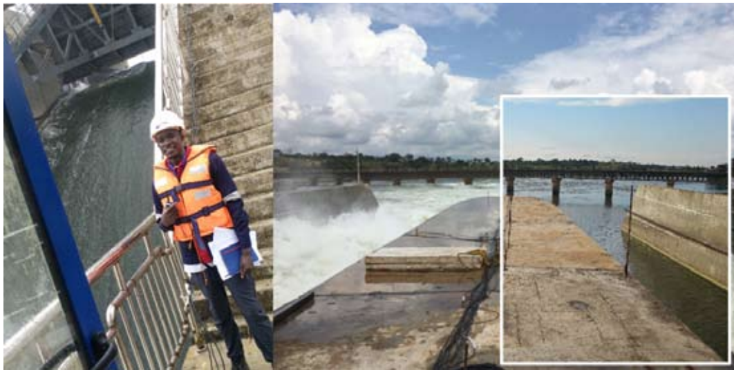
Figure 9 : Showing the right opening at 70% opening with the corresponding downstream water level rise
