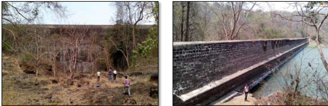
Figure 5 : Locations of Geophones at the downstream face and upstream face of the Tulsi dam No.1
