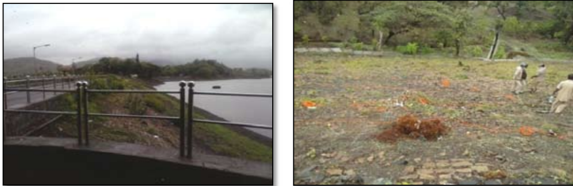
Figure 11 : Locations of Geophones at the downstream face, upstream face of the Vihar dam (Central Portion)
