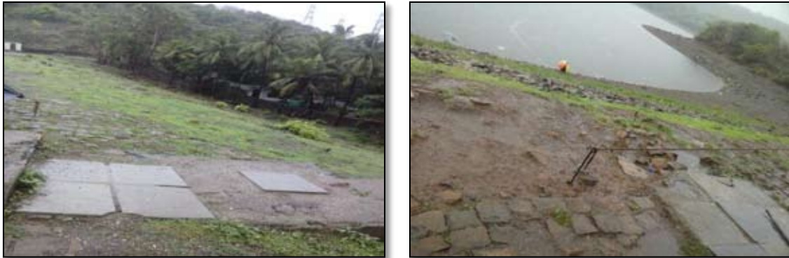
Figure 13 : Locations of Geophones at the downstream and upstream faces of the Vihar dam near Durgah
