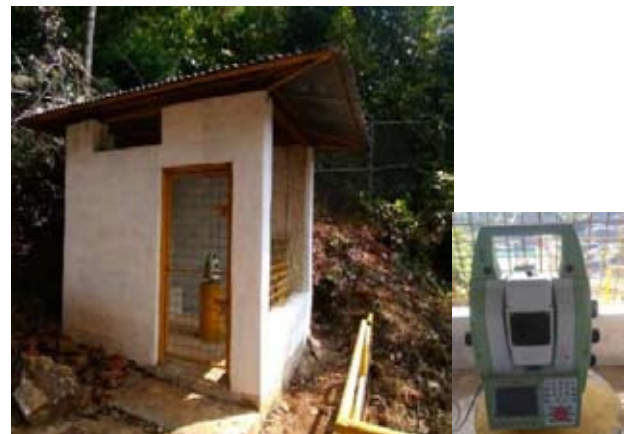
Figure 11 : Robotic shelter position
