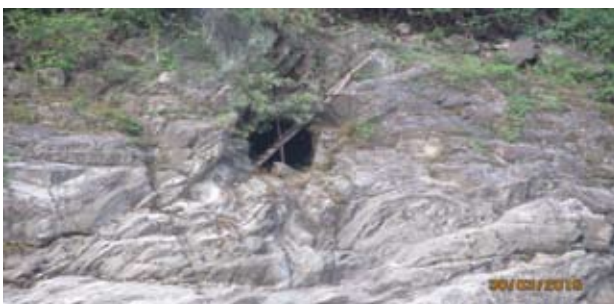
Fig 11 : Exploratory drifting in round 2 at dam area.
