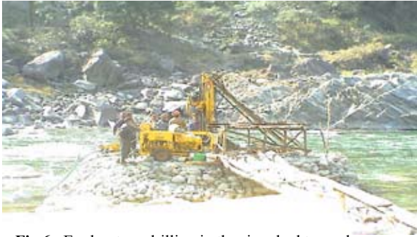
Fig 6 : Exploratory drilling in the river bed to explore dam foundation condition.
