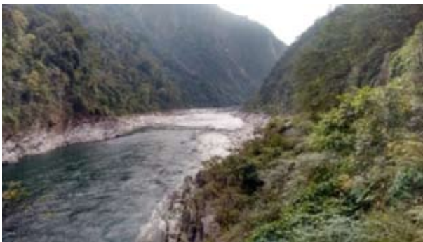
Fig 3 : Downstream view of the dam axis-III.
