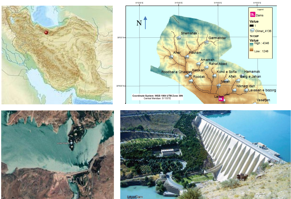
Figure 2. Site Location of Latian Dam
