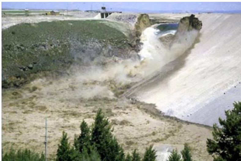
Figure 2. Failure of Teton Dam (Idaho) from seepage (1976) [2]
