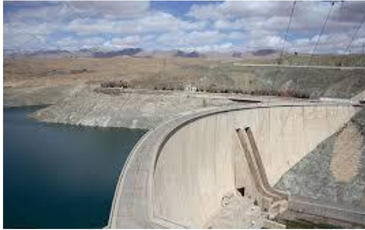
Figure 1. ZayandehRud arch dam
