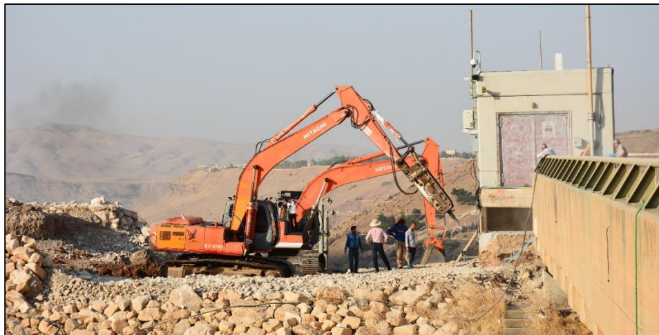
Figure 12: Excavation next to the spillway wall.
