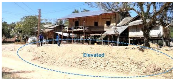
Photo 4. Residence elevated by Structural Columns (Wooden structural columns are seen under the house. Private land was also elevated by embankment.)
