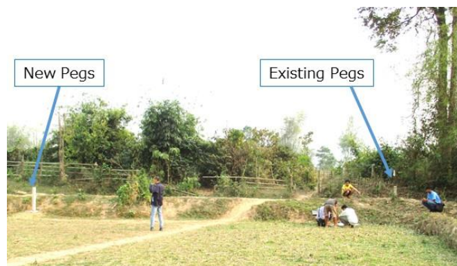
Photo 3. Re-Installation of Pegs (A new peg is seen in left side of the photo. On the right side PAPs are checking its position based on the map. An existing peg was seen on the right side as well, which was originally installed in the lower step but shifted by PAPs to the upper step so as not to interfere with cultivation.)
