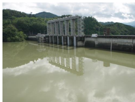
Figure 3. Photo of dam reservoir after the July 2018 flood
